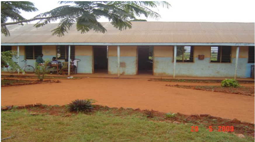
Figure 2: Classrooms Constructed at Vikenge Primary School
